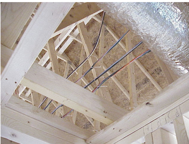
Runs of HYBRID (Fiber, CAT5e, CAT6, RG6 Q coax)
